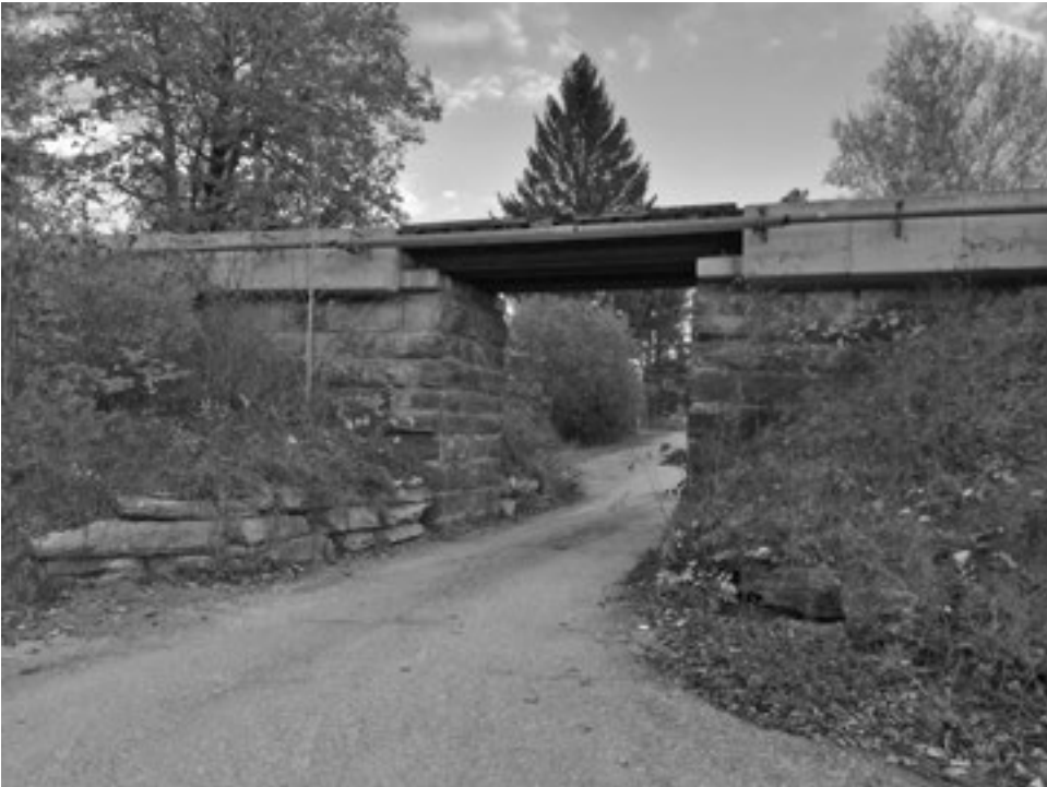
Original 1848 culvert off Bostwick Road in Shelburne, Vermont. The stonework, which is virtually identical to the underpass in New Haven, identifies it as original.
