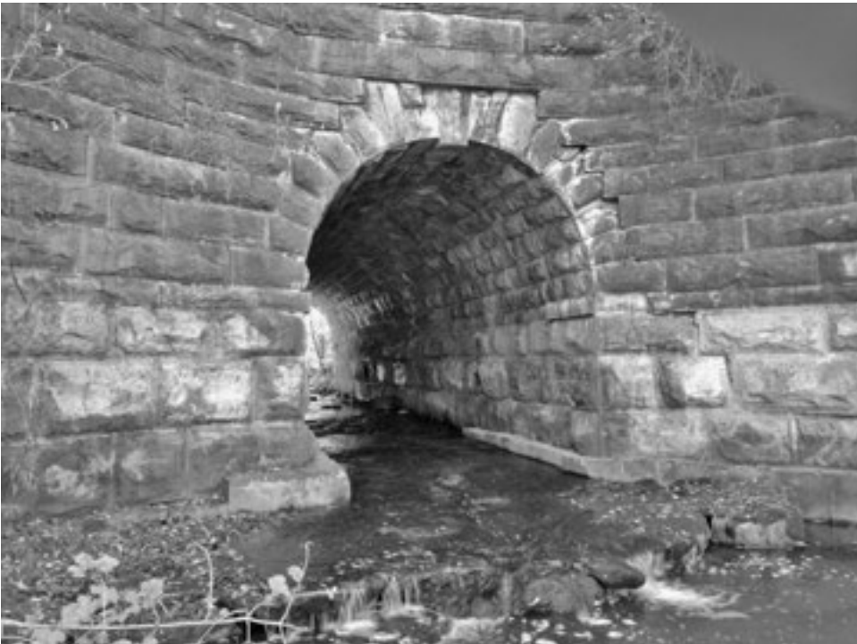
Original 1848 underpass on Belden Falls Road in New Haven, Vermont. Note the stonework, which is what identifies it as original. The cement section over the top occurred when the rail bed had to be raised for more road clearance.
